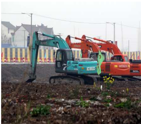
Shanghai Disney removal of potentially contaminated soil
